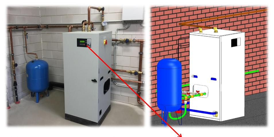
To keep a constant waterpressure there are 2 pumps fitted in the device with a steel enclosure. The system controls the entire rainwater system, including automatic filtercleaning.
