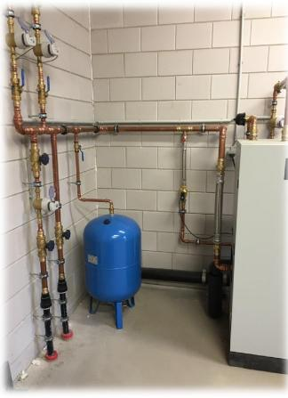
A commercial building equipped with a rainwater system. The rainwater is harvest from a roof of 1.500 m<sup>2</sup>. The rainwater is filtered and stored in a tank of 20.000 liter. This filtered rainwater is used for toilet flushing.
